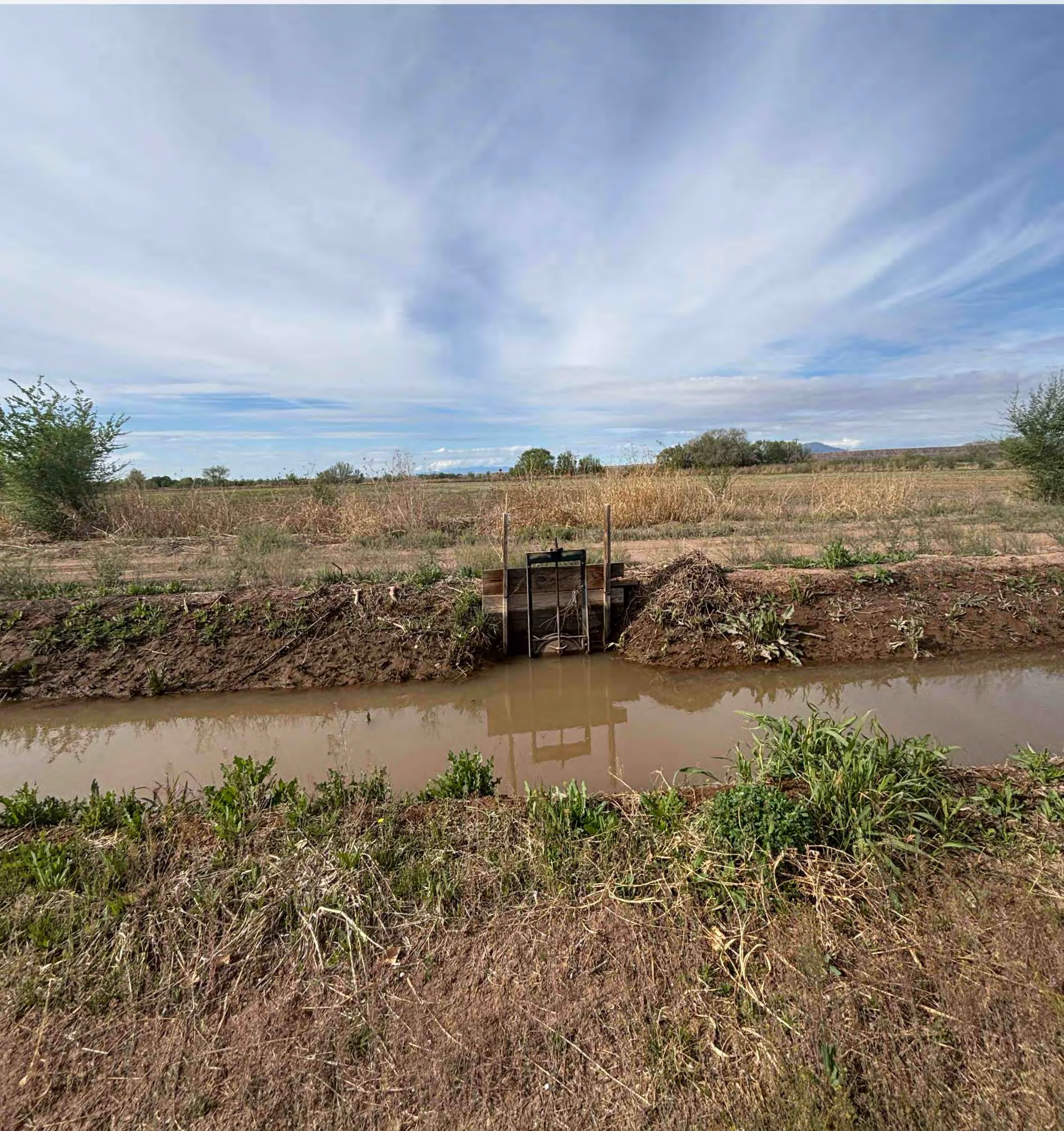
Photo 2, Turnout that supplies the southern half of Tract 18A1B.
