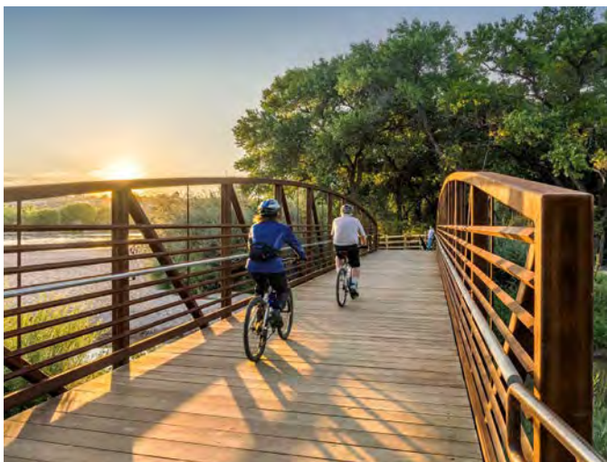
Bridge near the Paseo del Bosque Trail, Albuquerque Source: Dekker Perich Sabatini
