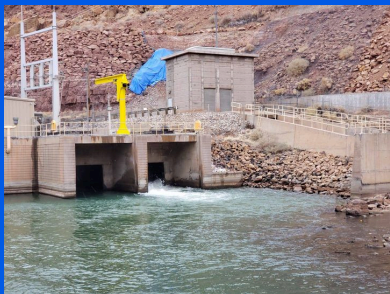
Outlet works at Abiquiu Dam: Photo courtesy of USACE
