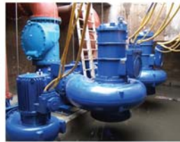
Submersible Pump and Motor Assembly
