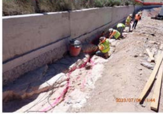
2023 – Slush Grout & Lean Concrete
