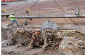
2023 – Concrete Saw Cutting
