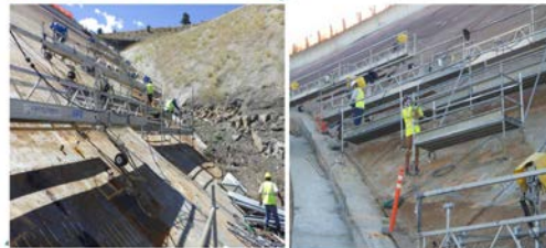
2023 – Backfill Grouting
