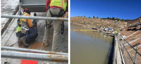
2023 – Backfill Grouting
