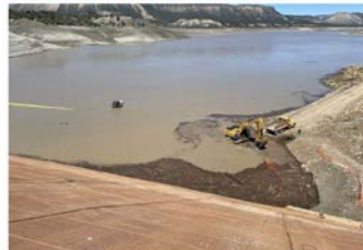
2023 – Outlet Debris Removal
