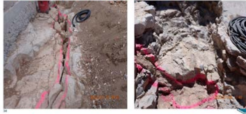
2023 – Slush Grout & Lean Concrete
