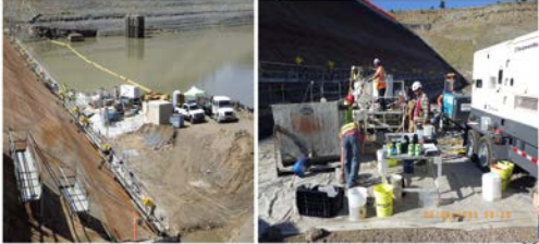
2023 – Backfill Grouting
