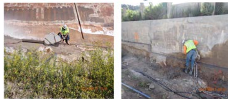
2023 – Concrete Saw Cutting
