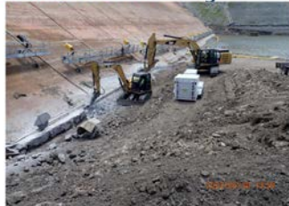
2023 – Plinth Wall Crack Repair
