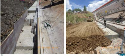
2023 – Slush Grout & Lean Concrete
