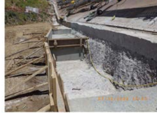
2023 – Slush Grout & Lean Concrete
