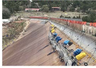
2023 – Slush Grout & Lean Concrete
