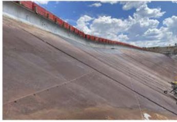
2023 Construction – Bulge Repair
