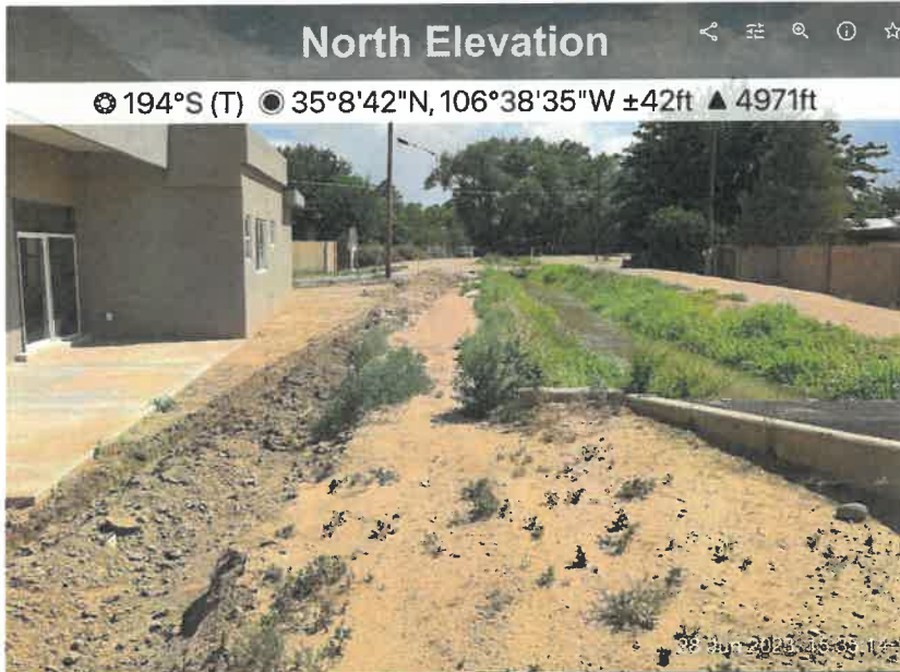
Figure A. Outer easterly edge of the ditch bank has been removed.
