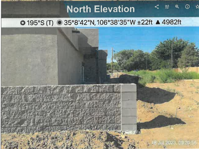
Figure B. Extent of block wall constructed as of July 18, 2023.
