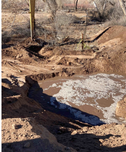
Corrales Siphon Sink Hole, East Side, 2022
