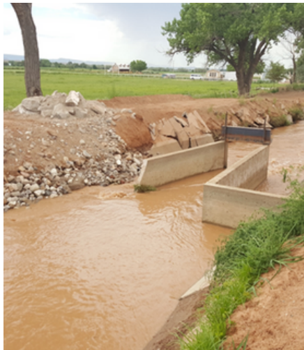
San Juan Main, Failed Long Crested Weir, 2016
