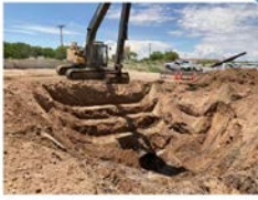
Isleta Interior Drain at Hwy 147, Temporary Repairs 2021
