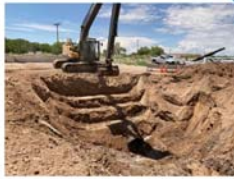
Ilieta Interior Drain at Hwy 147, Temporary Repairs 2021
