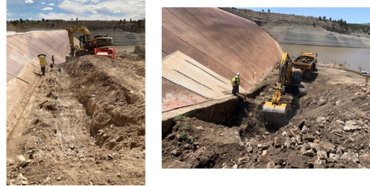
Construction: Excavation – Left Abutment
