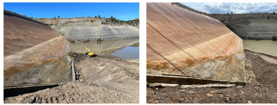
Construction: Excavation – Left Abutment
