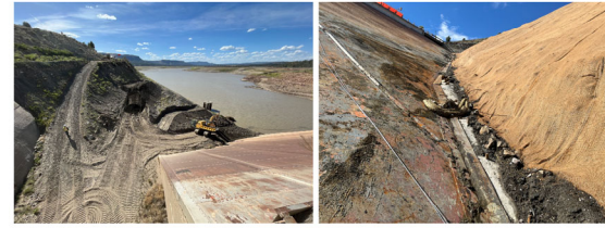
Construction: Excavation – Right Abutment
