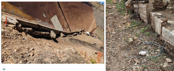
Differing Site Conditions Concrete Plinth and Cutoff Wall Geometries
