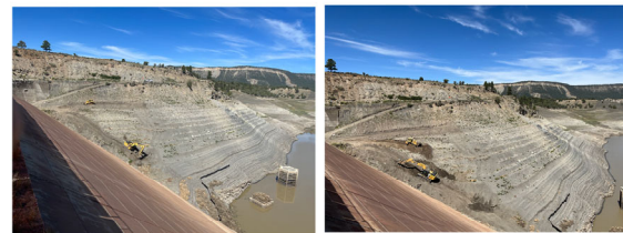
Construction: Excavation – Right Abutment
