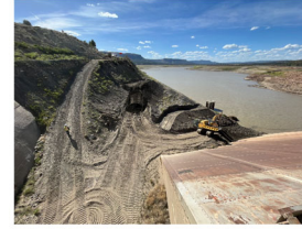
Construction: Excavation – Right Abutment
