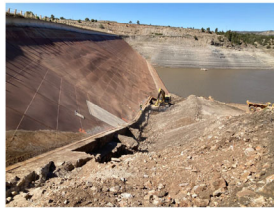
Construction: Excavation – Left Abutment
