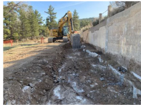
Construction: Excavation – Left Abutment
