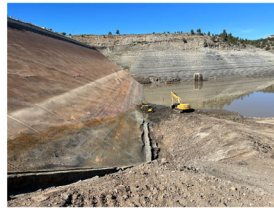
Construction: Excavation – Left Abutment
