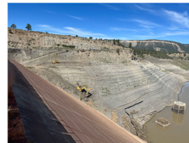
Construction: Excavation – Right Abutment
