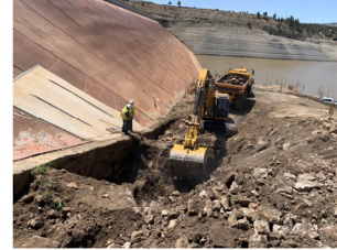
Construction: Excavation – Left Abutment
