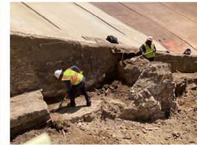
Construction: Excavation – Left Abutment
