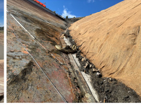
Construction: Excavation – Right Abutment
