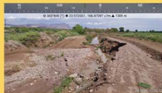
San Antonio Ditch ±86+00
