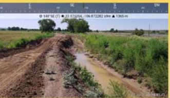
San Antonio Ditch ±92+00
