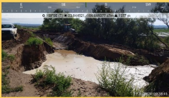
San Antonio Ditch ± 195+00
